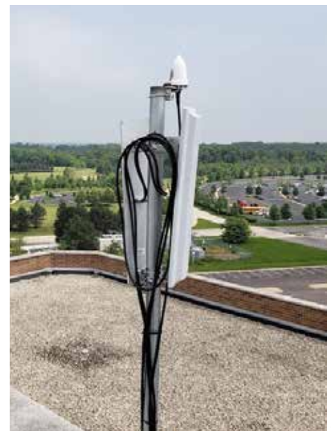
CBRS 3.5 GHz MIMO equipment installed by ExteNet.
